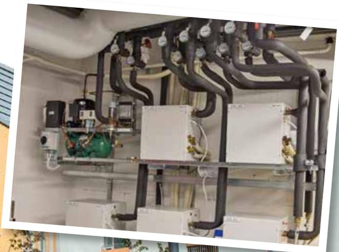
supplying the necessary condensation capacity for technical rooms, cold rooms, and the kitchens. A water-glycol solution circulates in the liquid cooling network. The technical rooms and cold rooms in the kitchen are cooled by DX fan coil units. The DX system is liquid-cooled and condensation takes place in the liquid-cooling network.
