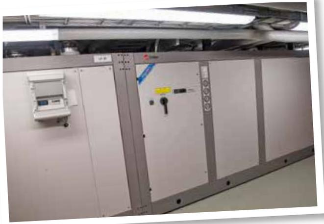
▶ **The geothermal energy of heating and cooling is produced by Chiller's heat pump; on cooling part by free cooling function. District heating works for back-up and auxiliary heating.**
